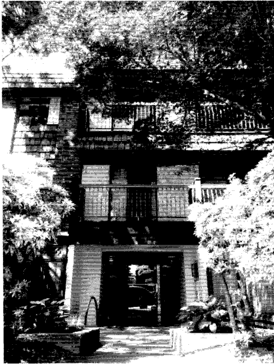
Figure 1 The main entrance to Twelve Oaks, May 2017. (Photo credit: Özgecan Yazar, used with permission.)
